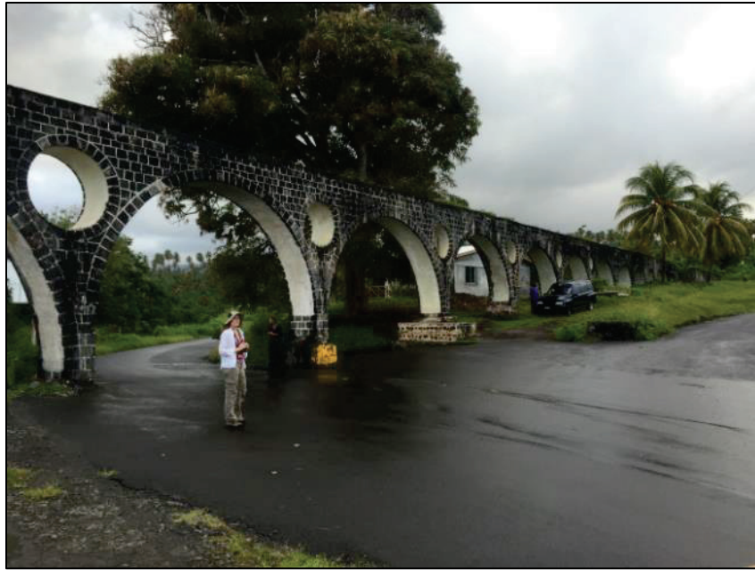
Figure 4-57: Orange Hill Aqueduct
