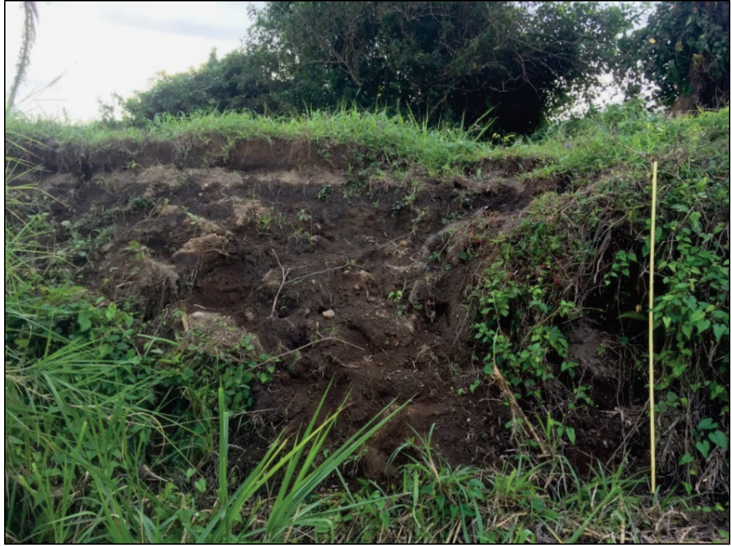
Figure 4-51: Orange Hill 1 Road Cut
