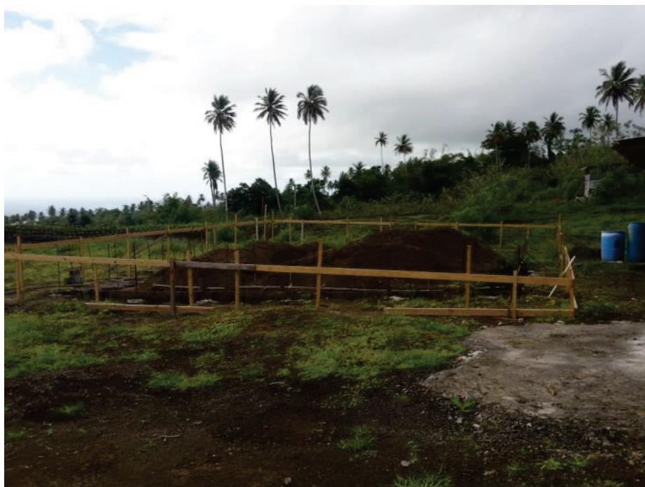
Figure 5-11: New Relocation Site
