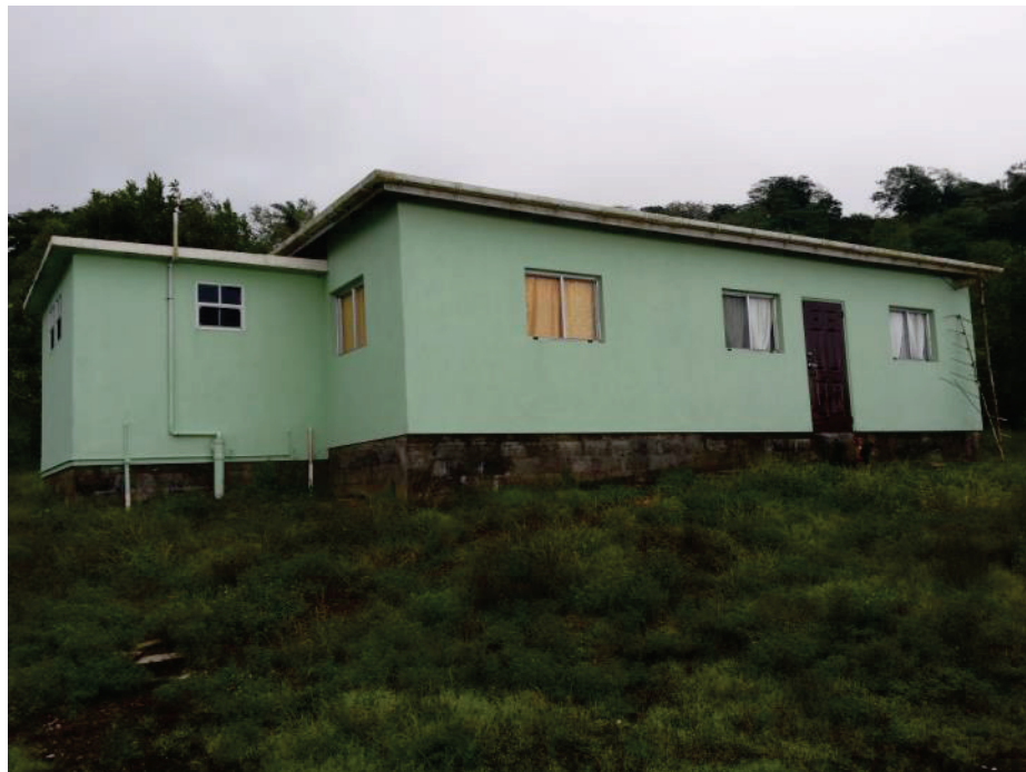
Figure 5-10: House to be Relocated
